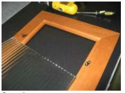
**Step 9** - Carefully insert glass avoiding contact between glass and metal clips.
