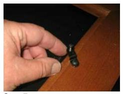
**Step 7** - After installing all metal clips swing the adjustment screws to the side to give you room for the glass to be inserted.
